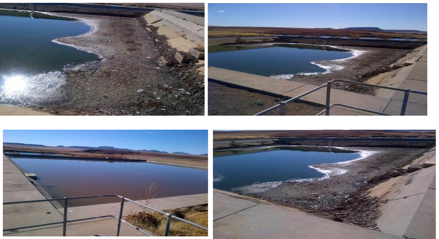
IMAGES ABOVE DEPICT THE SLUDGE BUILD-UP IN THE OXIDATION PONDS AND CURRENT PRACTICE OF EMPTYING THE PONDS TO ALLOW SLUDGE TO DRY FOR SAMPLING AND ANALYSIS
